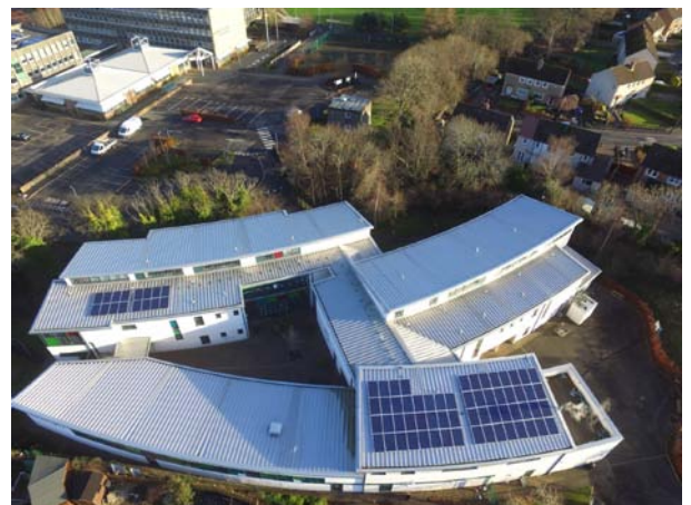
Solar Panels on Woodlands School (An Edinburgh Community Solar Co-operative Project)
